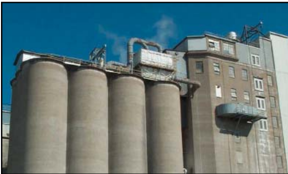
Donaldson Dura-Life filter bags, now installed in this Kice dust collector atop the elevator, are giving 4 times the life of the previous filter bags!
